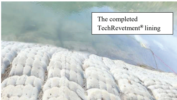
Fig. 7. The completed TechRevetment® mattress as seen from the surface
