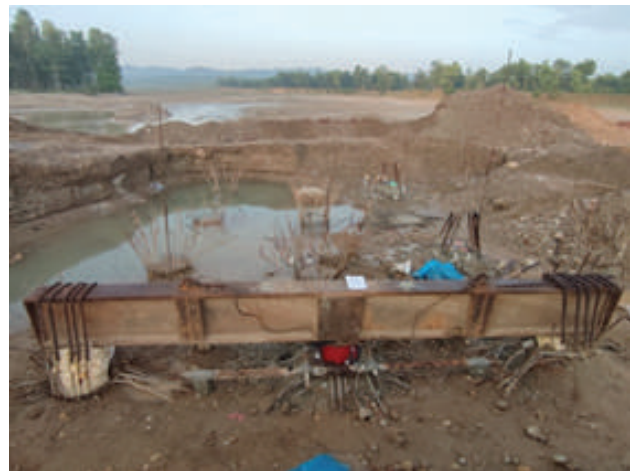
Figure 10: Static Pile Load Test (Anchorage Method)
