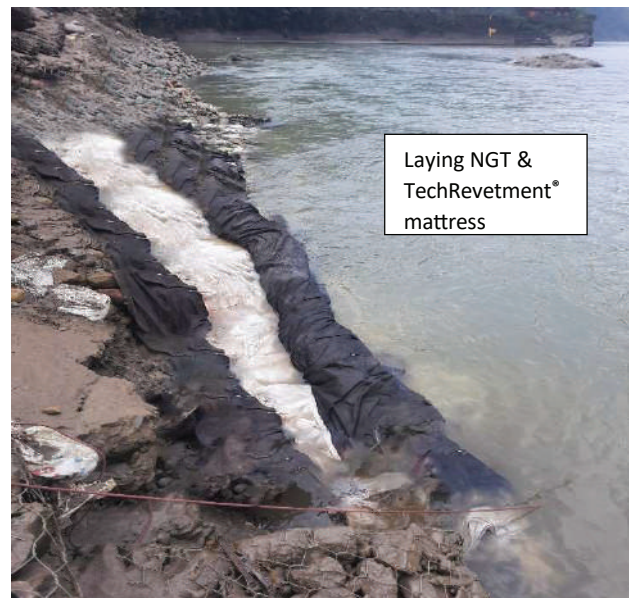
Fig. 5. Laying of NGT and TechRevetment® mattress
