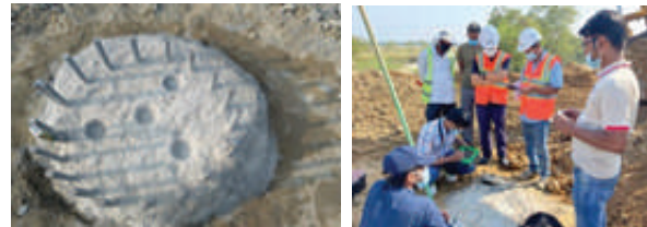
Figure 8: Pile Integrity Test (PIT)
