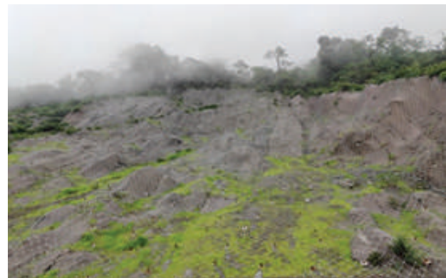
Figure 1: Narendranagar Landslide on completion
