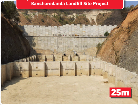
Nepal's Tallest Reinforced Earth® Structure at Bancharedanda Landfill Site Project
