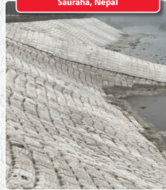
TechRevetment® Technology for River Bank Protection at Sauraha, Nepal
