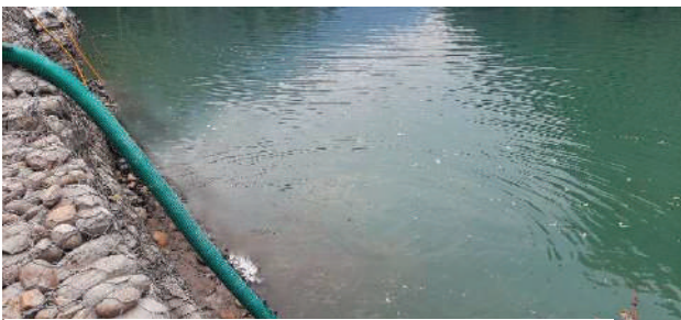
Fig. 4. Restoration work underway
