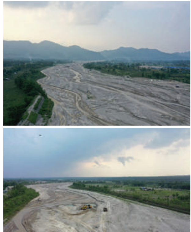
Figure 5: Aerial view of Bakra River showing aggraded river bed and mining
