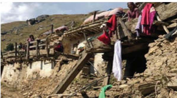
Figure 1: Infrastructure damaged due to disaster
